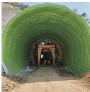
Fig NO- 5 Water proofing Installed temporary
