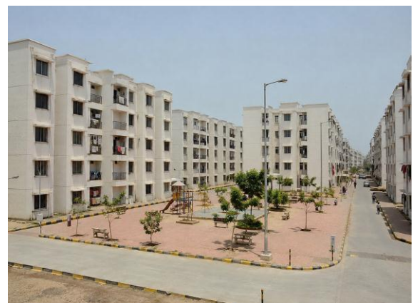
Figure 4: Rehabilitation Housing Blocks at Resettlement Site
