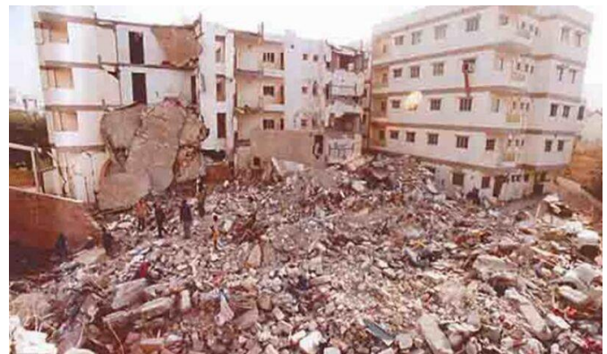
Figure 1 Damage caused by an earthquake
